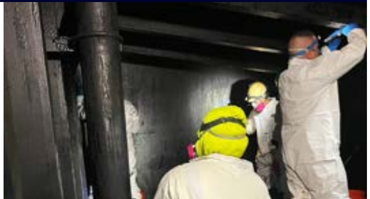
Cleaning Fuel Tank To Perform Repairs
