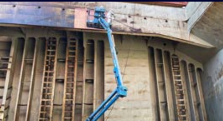
Cargo Hold Cleaning
