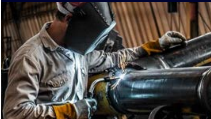
Pipe Spool Fabrication
