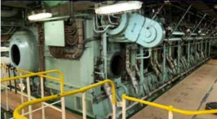
Piston Inspection Ports
