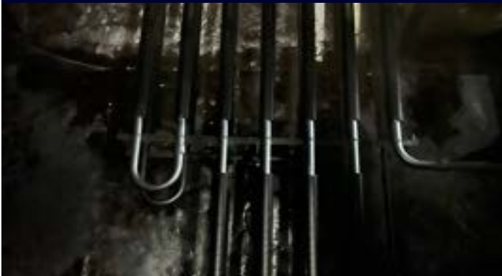
Steam Coils Inside Settling Tank
