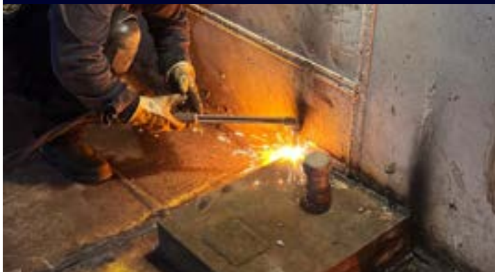
Ballast Tank Insert Repair
